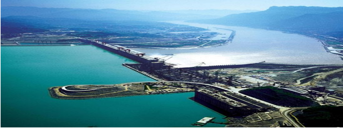
Fig. 1: Three Gorges dam of China the world’s largest power station [7]
